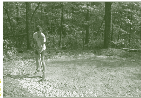
Elizabeth Pratt leveling gravel and dirt for an Earth Foundation Yome.
