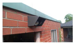
**Figure 1** | Light shield applied to an outdoor lighting fixture. Light shields, such as the one pictured above, can be very effective in redirecting excess light that could contribute to skyglow. The light is directed downward onto the surfaces it is intended to illuminate.
