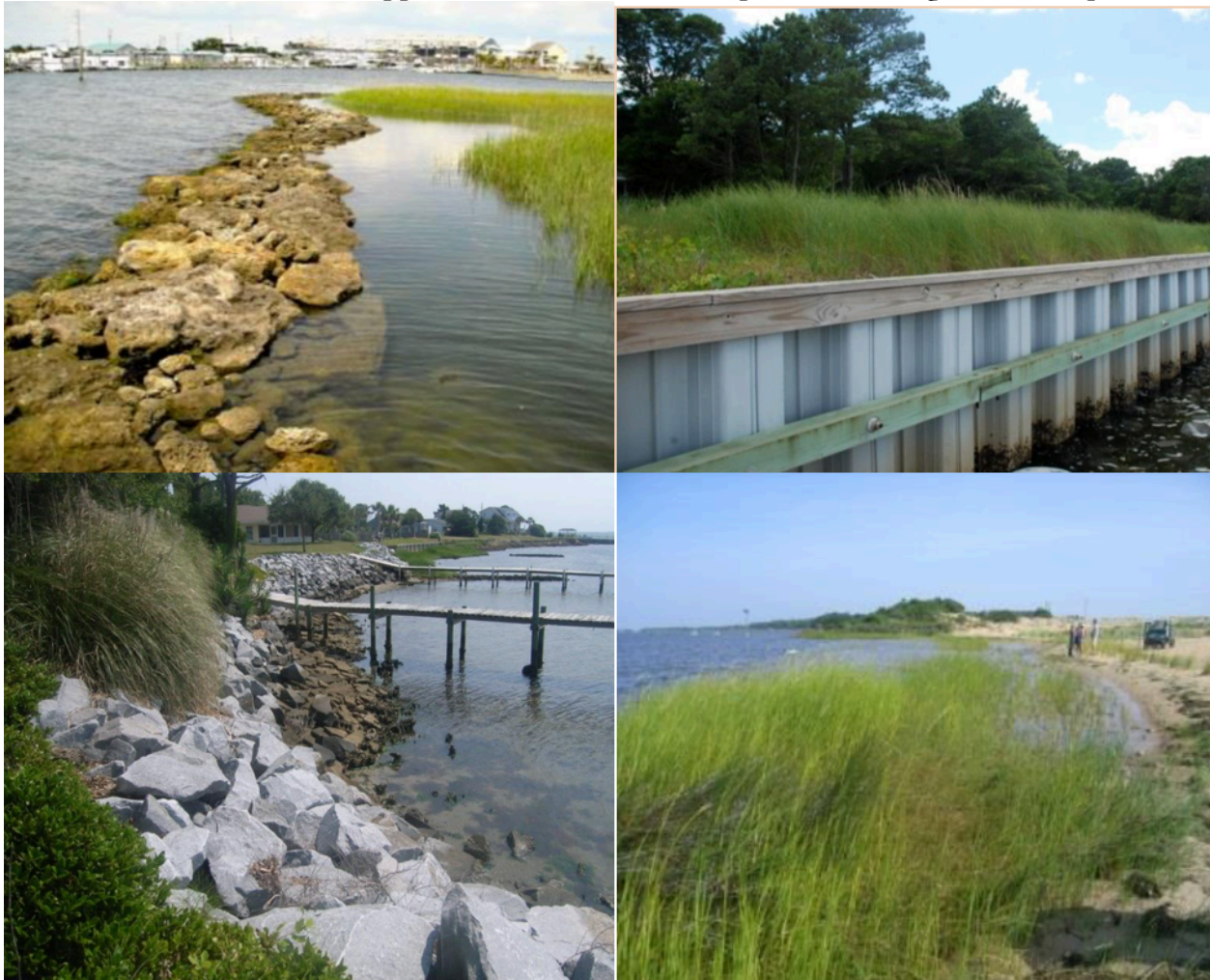
Figure 1. Examples of estuarine shoreline stabilization options. A living shoreline composed of a seaward rock sill with planted vegetation (top-left), a bulkhead (top-right), a riprap revetment
