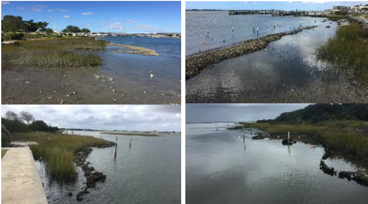
Figure 1. The four sites used by all groups for data collection. Top left: Continuous oyster sill at NOAA; Top right: Discontinuous oyster sill at UNC-IMS; Bottom left: Continuous granite sill at Duke University Marine Lab; Bottom right: Discontinuous granite sill at NC Maritime Museum
